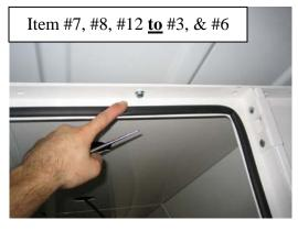
Continue around the entire kit bolting all **Ceiling** pieces to **Bulkheads** and **Doorframes** using ½ x ¾" carriage bolts, washers, and serrated nuts
